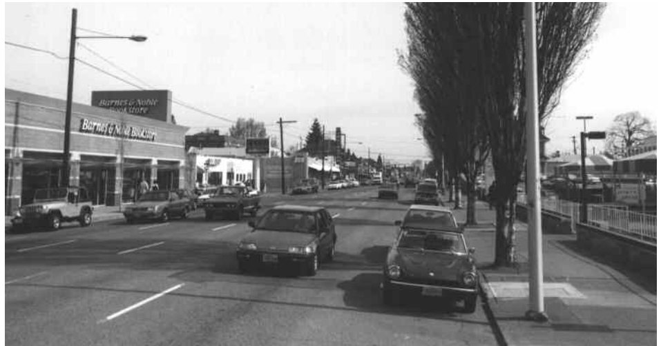
NE Broadway's four lanes would be reduced to three, retaining parking, and adding a bike lane. Narrow, upright trees like those on the right would be planted along the widened sidewalks. Parts of Weidler would have wider, spreading trees.
