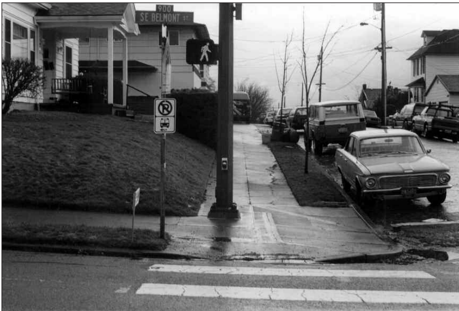
Newly installed pole at SE 50th and Belmont for a pedestrian crossing to a school. A preferred location would be in either planting strip.
