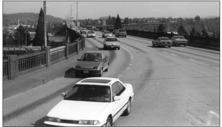
(Above) Ross Island Bridge from west end looking east. Only the north side of the bridge has a usable sidewalk. An open house on April 26 will be the first opportunity for public input on bridge plans. (Left) Detail of historic bridge railing.
