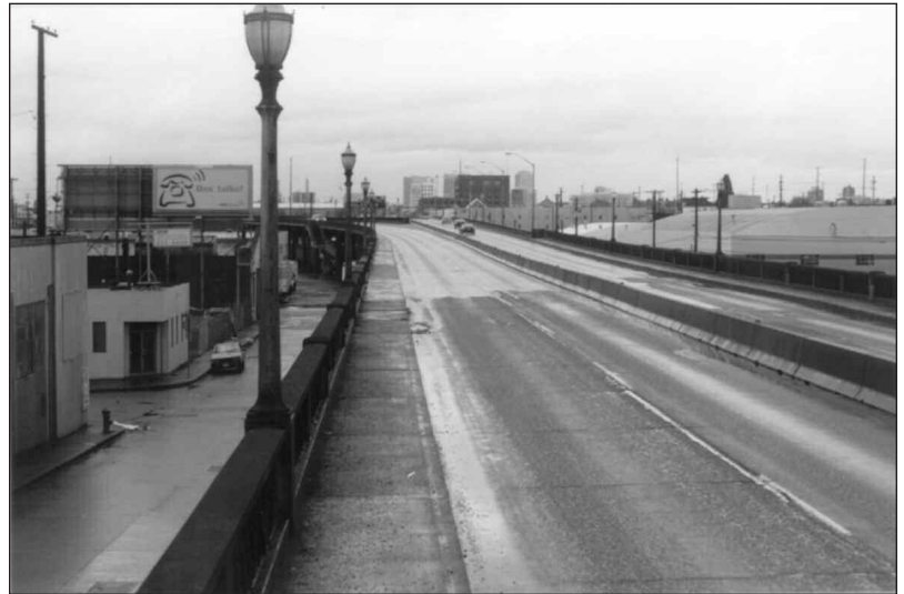
Looking north on the King-Grand viaduct from near SE Taggart Street.
